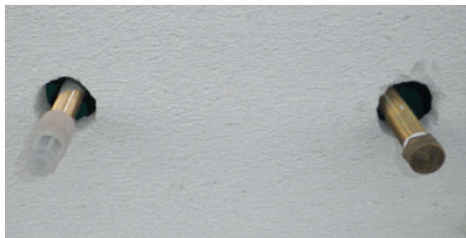
Figure 14.4 Neat finishing of installed services
