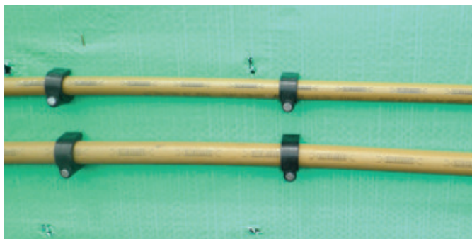
Figure 14.3 Install piping services prior to the installation of STAAC WALL® panel
