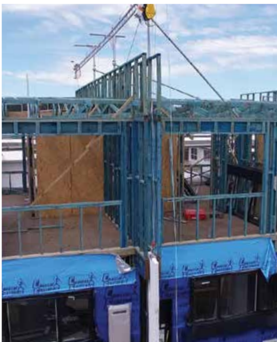
Figure 5.1 Hoisting of dual zero boundary wall in operations
